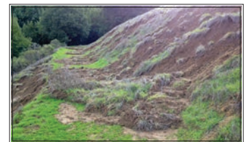
Dutra Ranch. Oversaturated soil slides downhill and obstructs trails.
