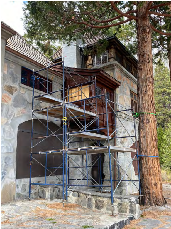
Restoration in Progress Funded by SSPF
